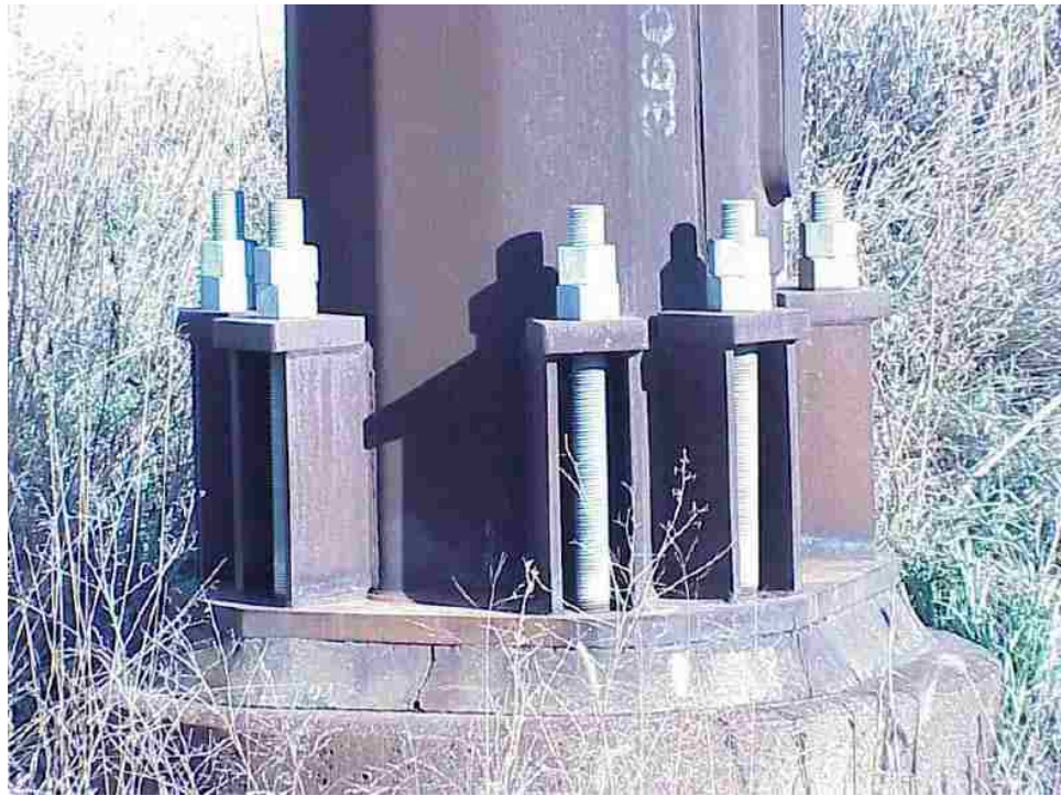
Figure 6. Stool base connection detail ( reprinted from Dexter, 2004 )
