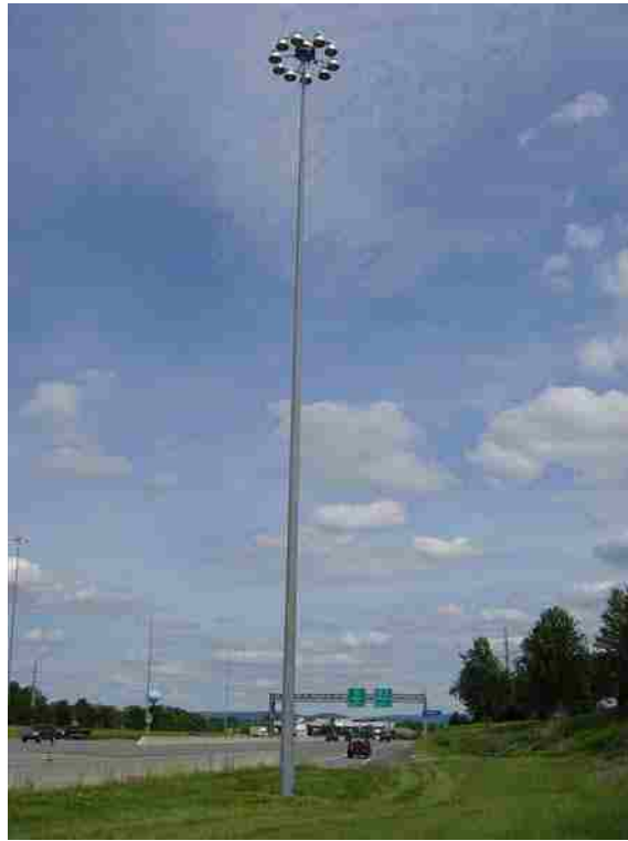
Figure 1. Example of a high-level lighting pole in service
